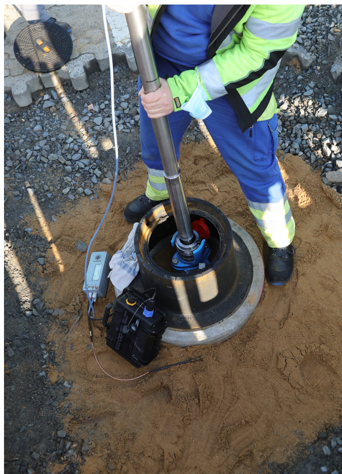
Trial installation of measurement lock
