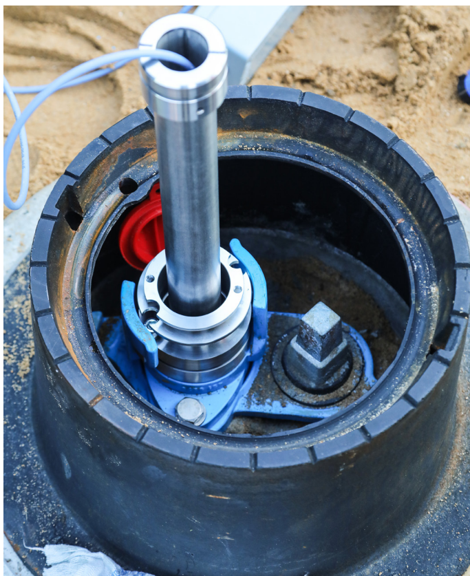
Trial installation of measurement lock
